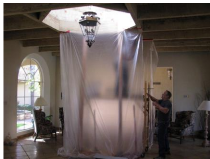
Repairs in Progress 1.7.10
