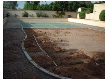
Construction photos. West court; work in progress. (August)
